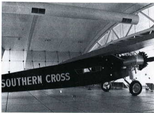
Moisture from this overhead supply duct has been falling directly onto the aircraft. The FAC has revealed that this is just one of several major conservation problems associated with the new Southern Cross enclosure.
